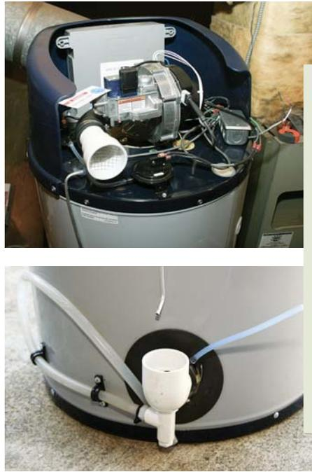
**Figure 3.** Condensing heaters can often connect to an existing 1/2-inch gas line. The plumber extends the line (far left) to reach the inlet at the top of the heater. The air intake (above left) — the PVC fitting with the screen inside — is connected to a draft-inducing fan. Combustion gas and condensate exit through a fitting near the bottom of the tank (below left). The elbow connects to the flue and the condensate hose runs to a drain.
