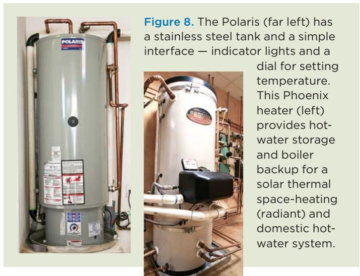
**Figure 8.** The Polaris (far left) has a stainless steel tank and a simple interface — indicator lights and a dial for setting temperature. This Phoenix heater (left) provides hot-water storage and boiler backup for a solar thermal space-heating (radiant) and domestic hot-water system.
