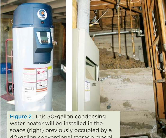
**Figure 2.** This 50-gallon condensing water heater will be installed in the space (right) previously occupied by a 40-gallon conventional storage model.
