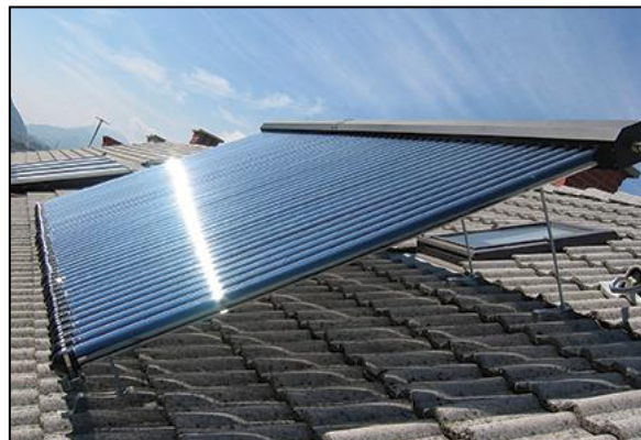
30-tube solar collectors from HTP have been certified by the Solar Rating and Certification Corporation (SRCC).
