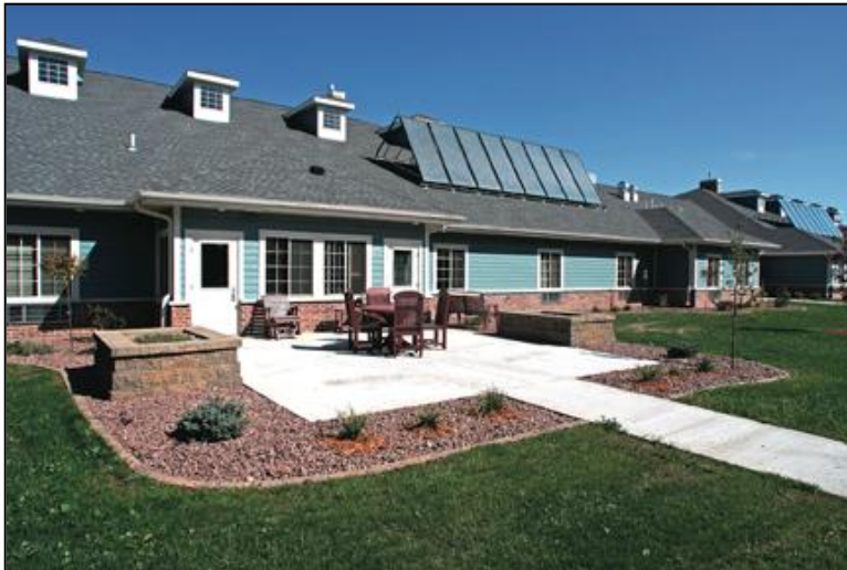
The Pine Ridge Colby facility (above) uses a solar thermal system to provide hot water to its in-floor radiant heating system, working in conjunction with the two Munchkin condensing boilers. The 16 solar collectors can be seen on the facility's rooftop in this photo.
