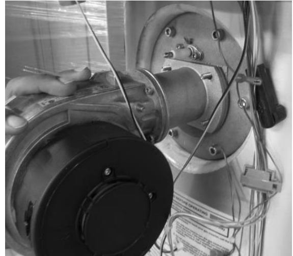
Figure 5 – Nuts and Washers Removed from Blower Assy
