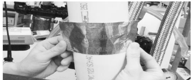
Figure 19 – Covering the Hole in the Exhaust Vent
