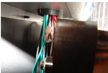
6. From the front of the boiler, feed the ground wire Up into the control box
