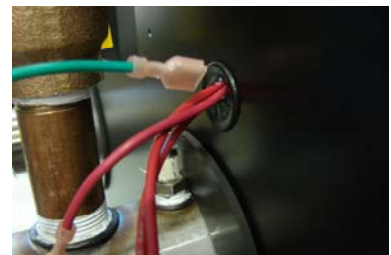
5. Feed Green Ground Wire into Boiler through the wire access
