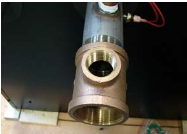
2. Thread brass Tee into outlet nipple using pipe dope.
